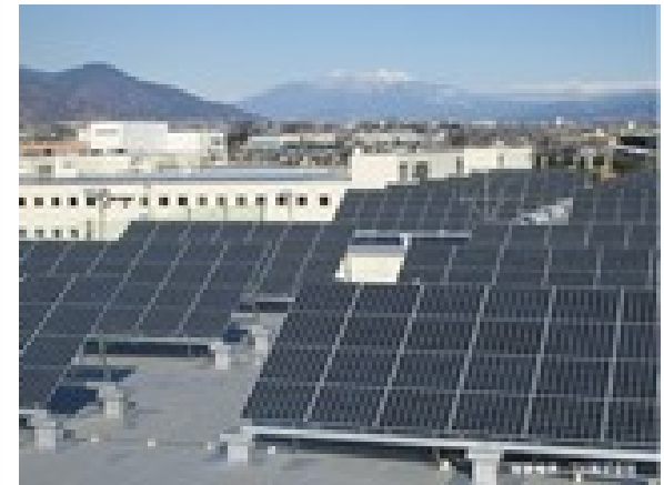
Large-scale solar panel installation on plant roof
