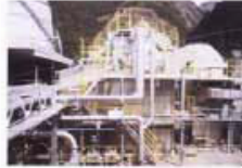
Wood Chip Burning Boiler
