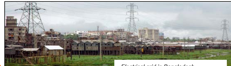
Electrical grid in Bangladesh
